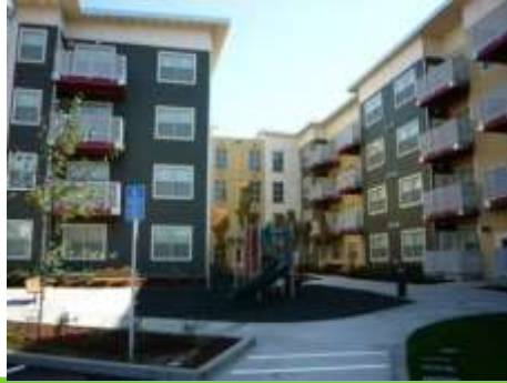
Esperanza Court, Portland (Catholic Charities Affordable Housing Project).
