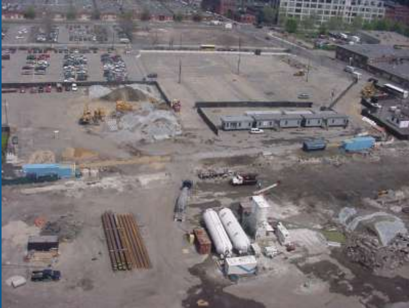
Former Manufactured Gas Plant
