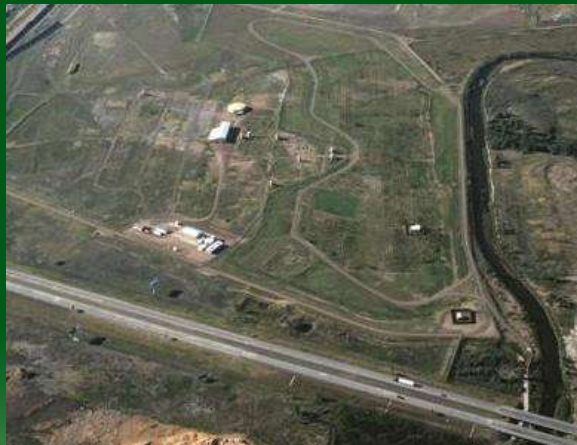
2004 – Former Wood Treating Plant – Creosote Recovery Completed
